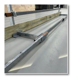
The unique design holds a consistent perimeter bump stop which alerts plant and equipment operators that they are near the perimeter guardrail system and helps prevent plant from coming into contact with the guardrail system.
